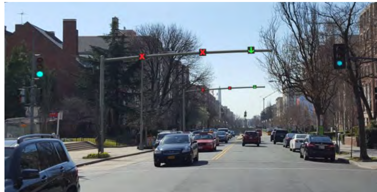
Overhead Lane Control Signs
